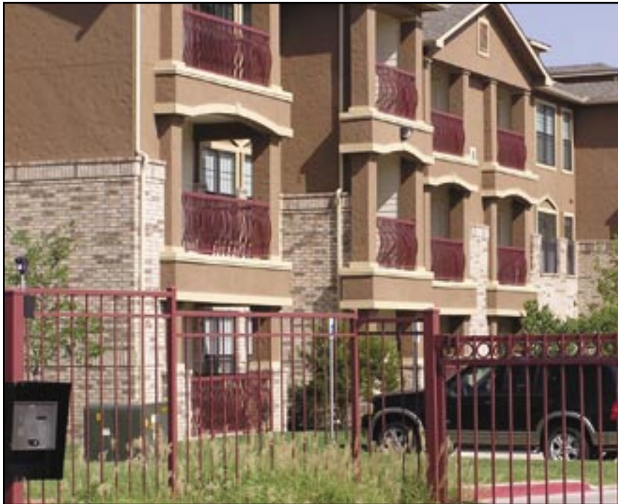
Even new builds, such as this property, can offer many unique service challenges.
