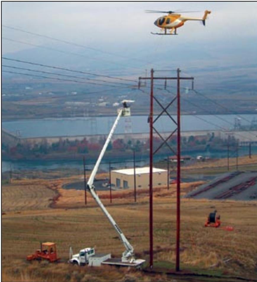
*Stringing fiber on a long tower-to-tower span in the Columbia River Gorge near The Dalles, Oregon.*
