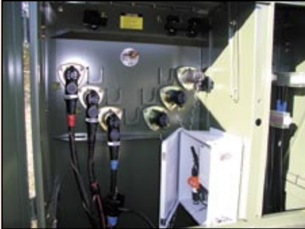
A typical fiber-to-powerline conversion point, installed in a pad-mounted transformer (left) and the E-PON Optical Network Unit (ONU) opened to see the inner workings (right). Each node location services anywhere from 10 to 40 customers with BPL service.
