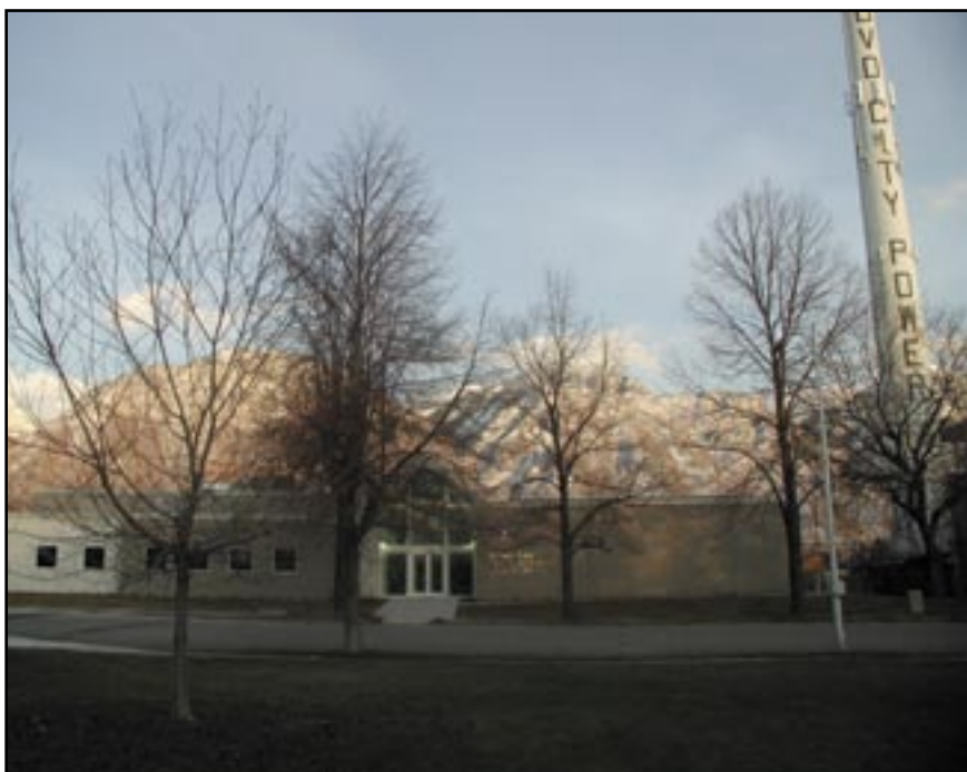
Provo City Power leases its headend, shown here, to the neighboring Utopia project. Utopia is also using Provo's satellite dishes. Provo is funding its project with a $39.5 million municipal bond.
