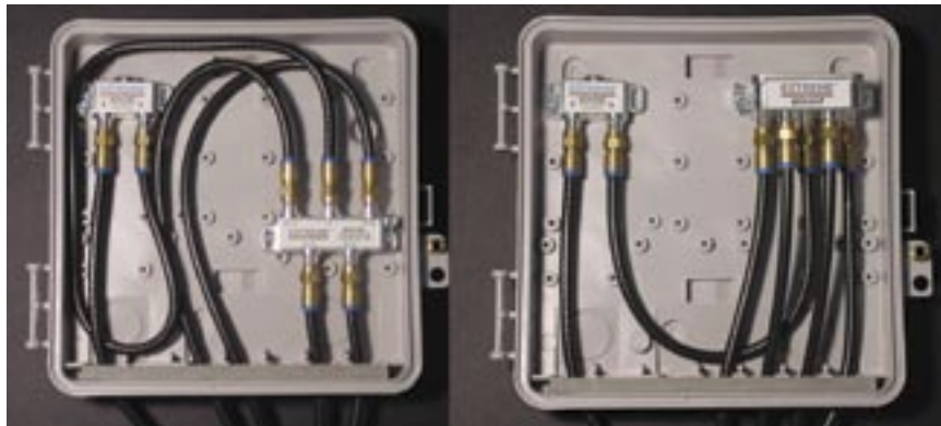
Left: Conventional splitter is a tight fit in a premise enclosure. Right: Vertical True Flex splitter reduces cable bends
