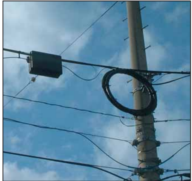
This weatherproof splice enclosure (Wave7 Last Mile Tap) is installed at the Taki-Cho project in Japan.
