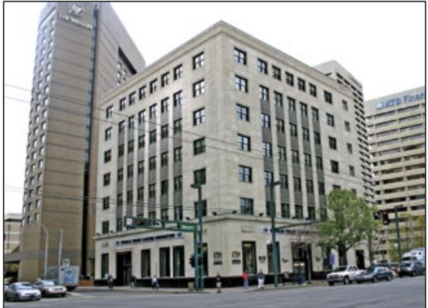
The new EEDC headquarters is in a historic downtown Edmonton building subject to traffic vibration, high winds, and harsh northern climate.
