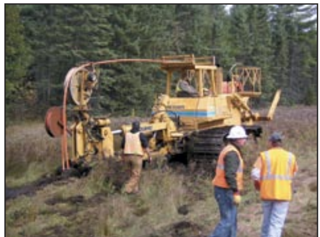
Deep trenching to lay fiber deep enough to keep weather, animals, and snowmobilers away.
