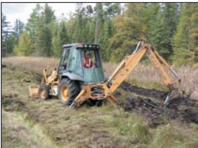
Deep trenching to lay fiber deep enough to keep weather, animals, and snowmobilers away.
