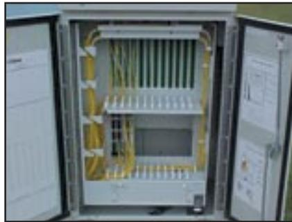
Pictures from Wakefield, a Horry FTTH community in Longs, SC, built by Beazer. About 150 homes are being served. A punchdown block in each home's garage carries CATV, voice and data. The cabinet at upper left can actually handle 216 homes. Horry Telephone Cooperative is also working with developers of larger communities.
