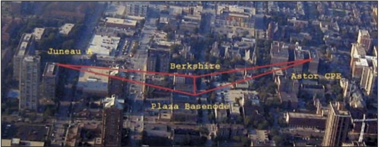
Figure 2. Four Omni-Nodes in a mesh configuration on four MDU properties in Milwaukee. Laying fiber in this congested area would have cost too much and taken too long. The saving over lease lines is $500 per line per month, giving a payback time of about eight months for the four-line solution shown here. Shoreline Real Estate owns 70 buildings in the area.
