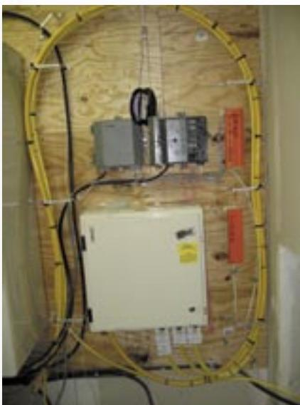
*At the Building Communication Gateway. Note the gentle bending radius of the fiber ducts.*
