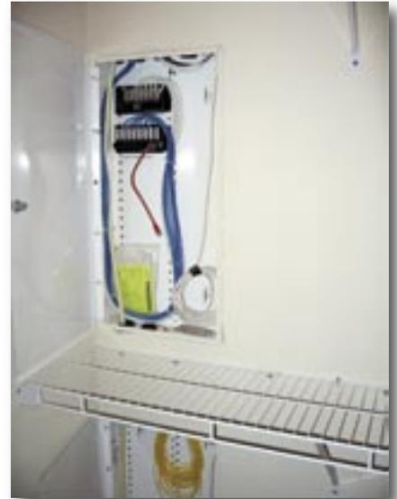
*Cabinet wiring before adding the battery backups and ONT.*
