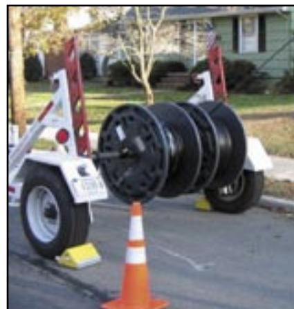
Figure 4: Preconnectorized aerial fiber comes off a conventional spool.
