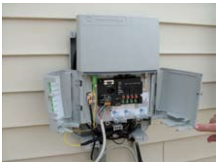
The ONT model chosen can output fiber, Ethernet, copper pair, and coax.
