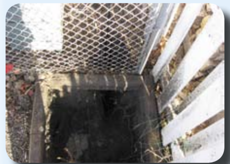
A hydrovac hole for a FTTH pedestal.
