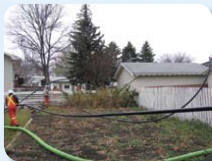
Preparing to pull conduit through a bore hole.
