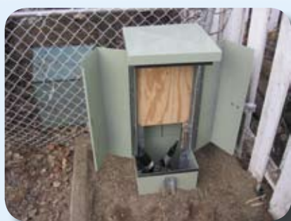
Steel pedestal placed with conduits.
