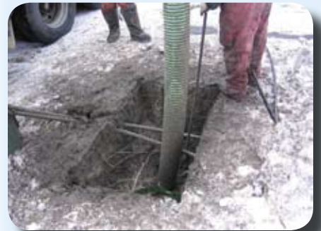
Using a hydrovac in a handhole.
