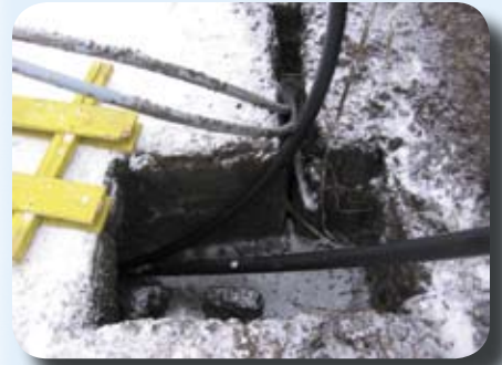
Directional boring in a customer's front yard.
