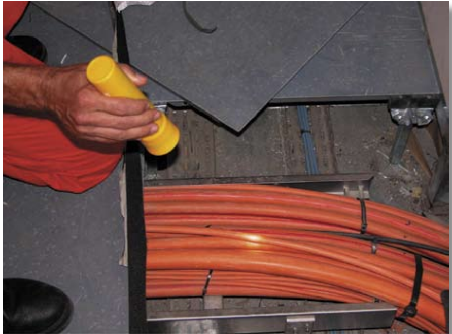
Ruggedized, tight-buffered cable derives much of its reliability and performance advantages from its basic design.
