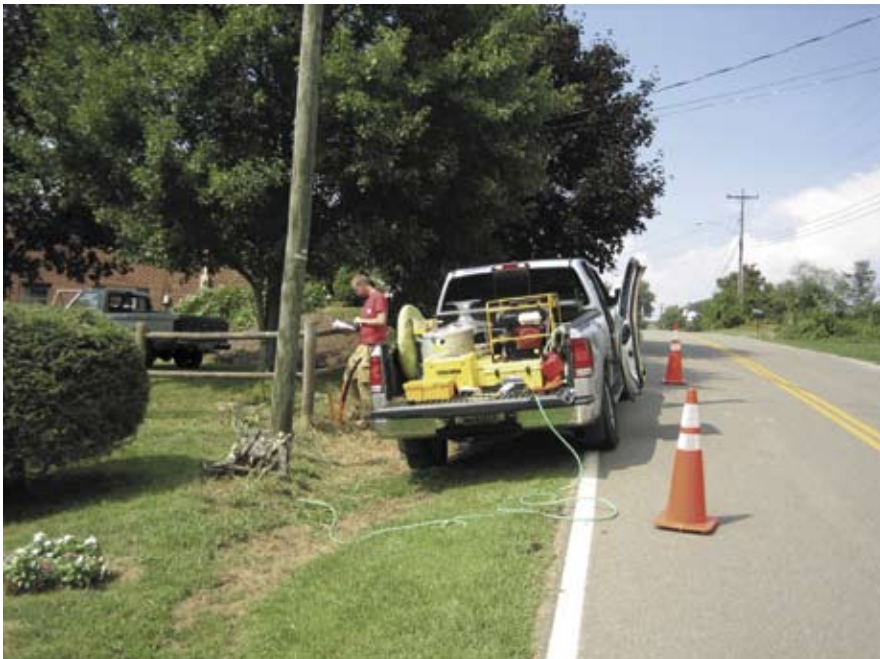
Figure 7. Blowing fiber into buried microduct to serve new customer.
