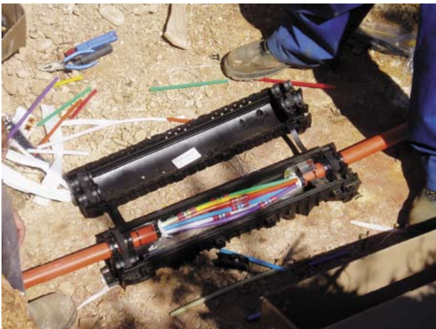
Figure 6. Splicing two lengths of multiple-tube microduct together in the field.
