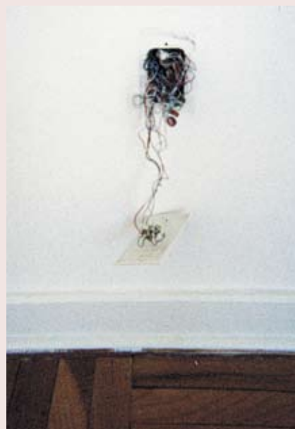
Legacy daisy-chained multiple pair twisted copper cable, unfit for almost any service.
