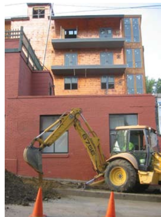
Bringing fiber to a multiple dwelling unit.
