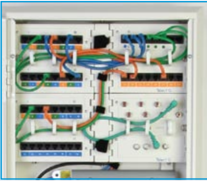
Closeup of the internal connectivity in a structured cabling panel. Color-coded ports and patch cords help to simplify installation and maintenance. Basic cable management ties keep the panel orderly and simple to access.
