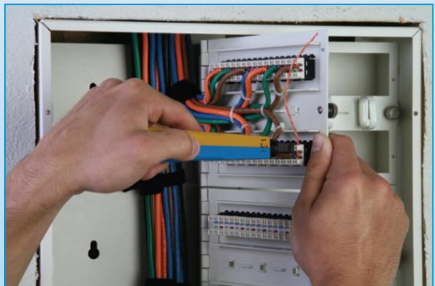
Module “carriers” inside the structured cabling panel pivot for simple installation and wire connection.
