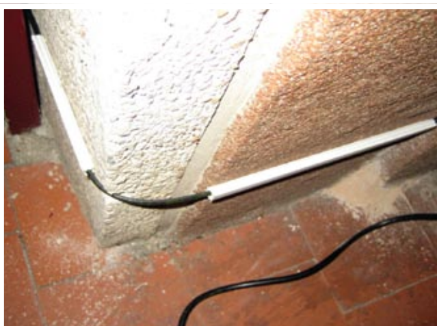
Figure 2. Path around corner; note the slight groove in the wall at corner bend.
